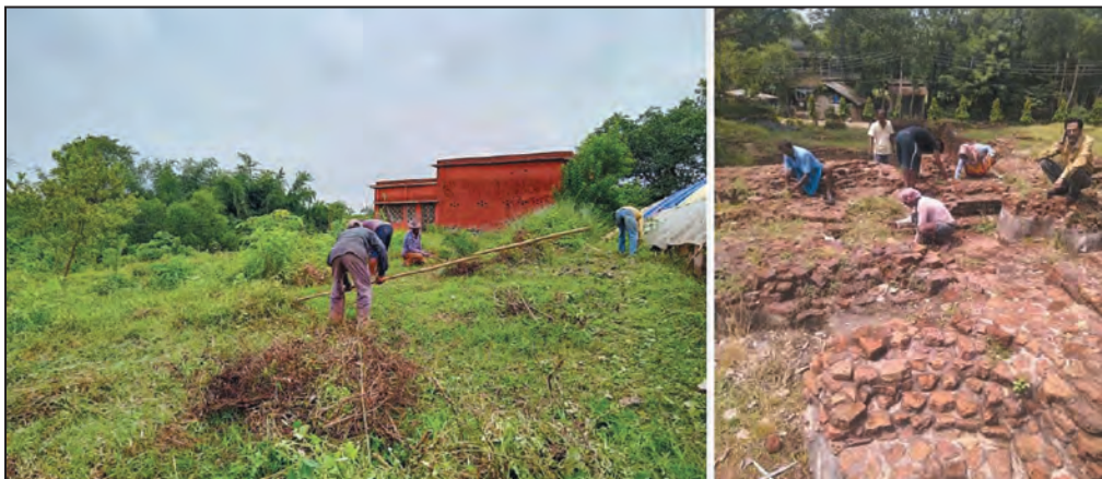
Fig-5 | Cleaning and clearing of site for work
